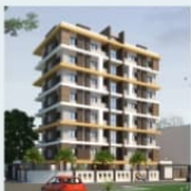
SHREE MANGALDEEP APARTMENTS
